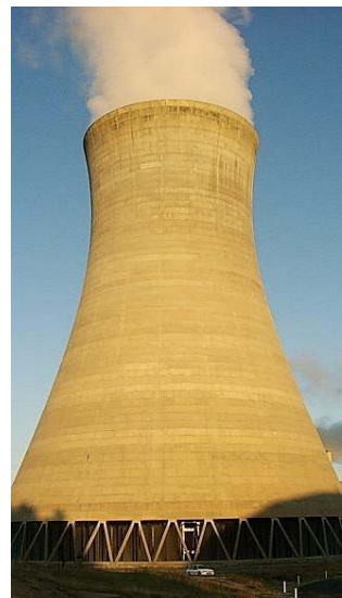
Wallerawang Power Station – concrete condition assessment
