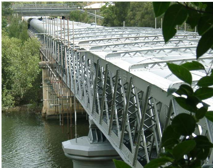
Wolli Creek Aqueduct – Lead Paint Management (specification and environmental monitoring)
