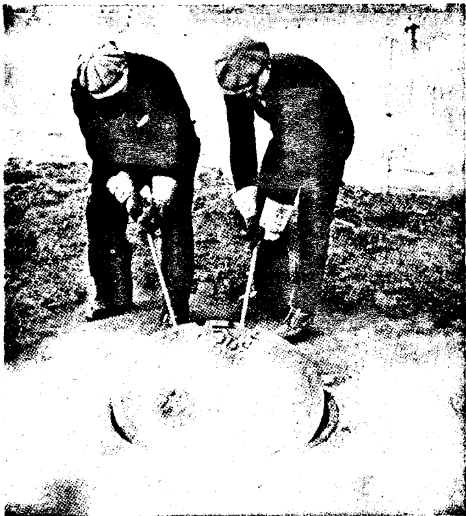
Removing Round Manhole Cover Using Manhole Bar and Manhole Hook
