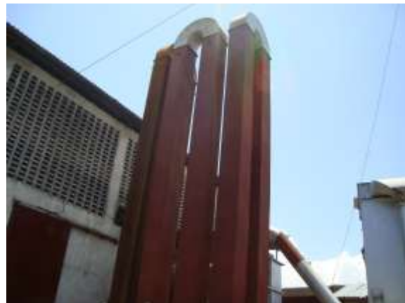
Lead filters of the factory
